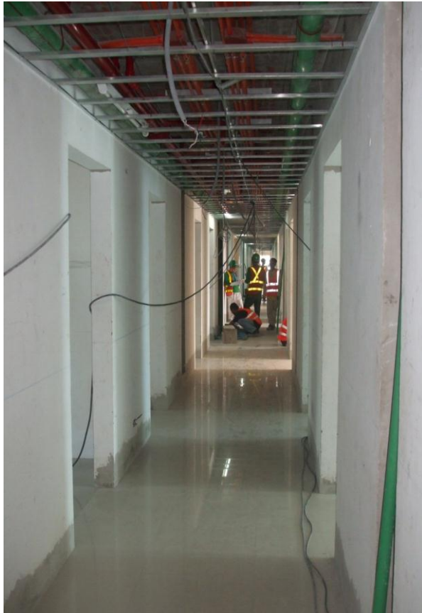
11 th Floor Hallway
